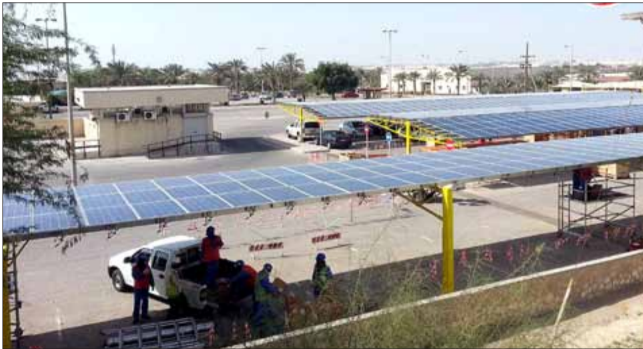
■ The solar panel being installed
